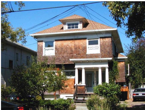
House: Residential endpoint of electricity.
