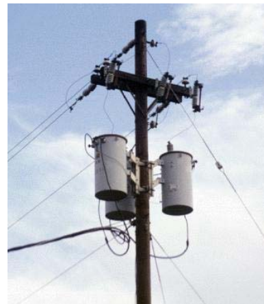
Transformer Drums: Convert electricity to lower voltage for use in a house.
